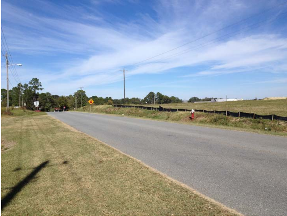
Figure 16: Water line on Seabrook Drive running down the west side of the property
