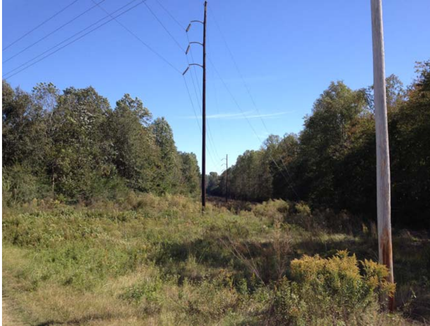
Figure 5: Power line easement running down the southern portion of the property.
