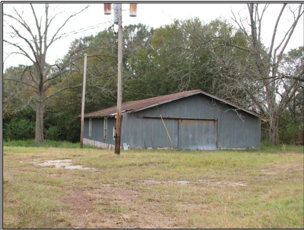
Photograph 21. View of Resource 6, associated workshop, northeast oblique.
