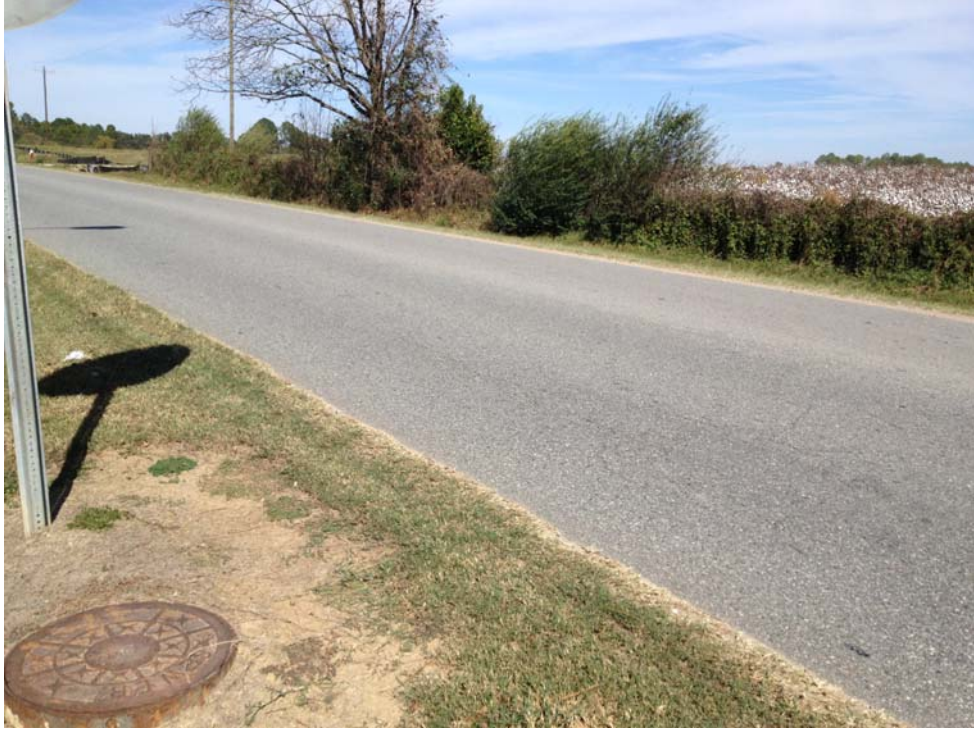
Figure 18: Sewer line located on Seabrook Drive with proposed site across the street.
