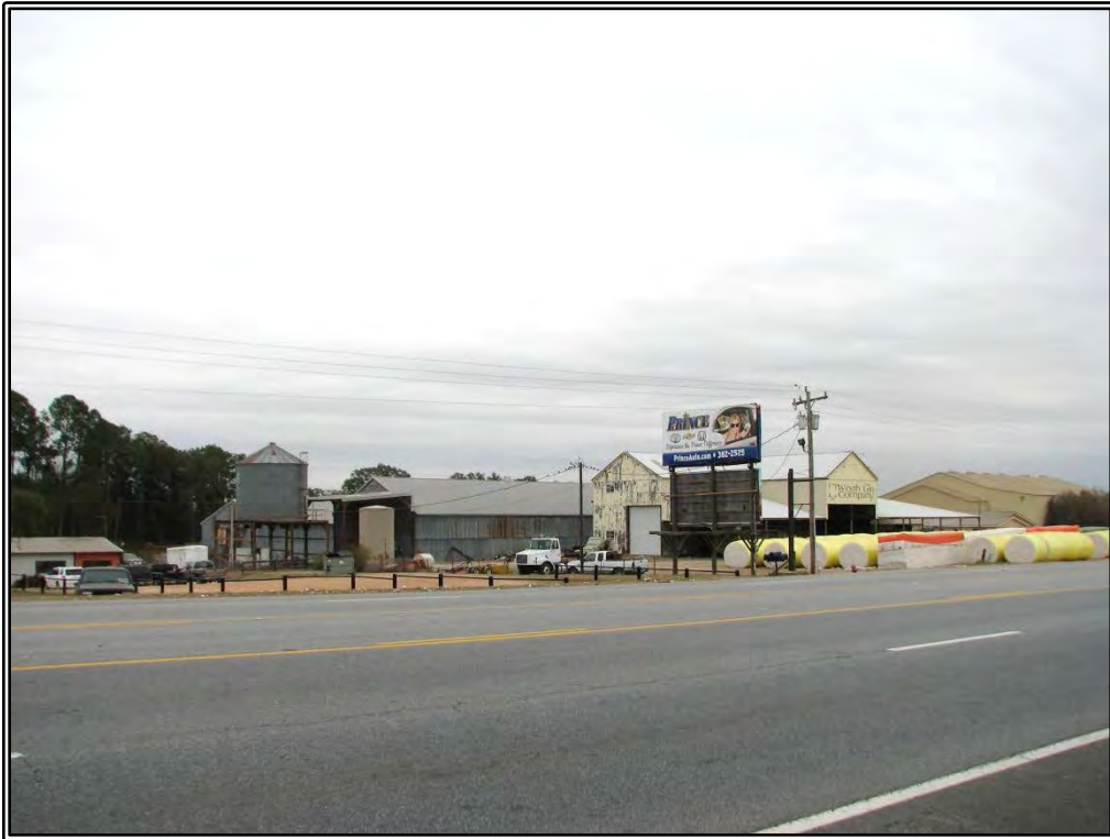
Photograph 15. View of the Resource 4 complex, looking northeast from US 82.
