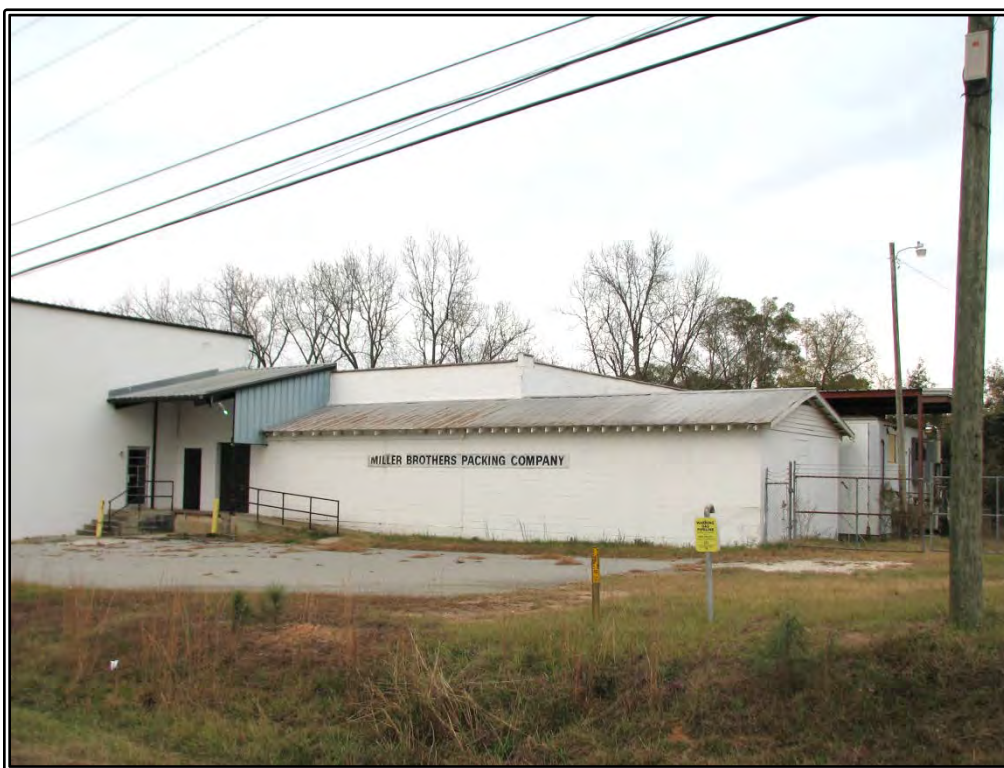
Photograph 19. View of Resource 6, northwest oblique, circa 1970 addition at left.
