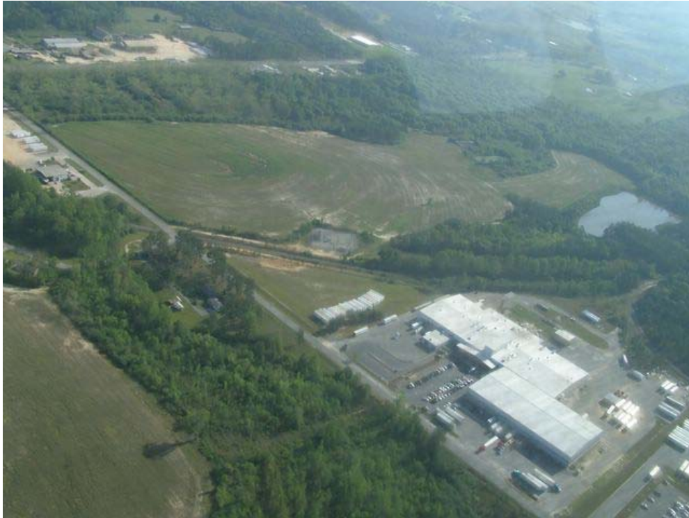
Figure 20: Aerial image of the proposed property looking to the northeast.
