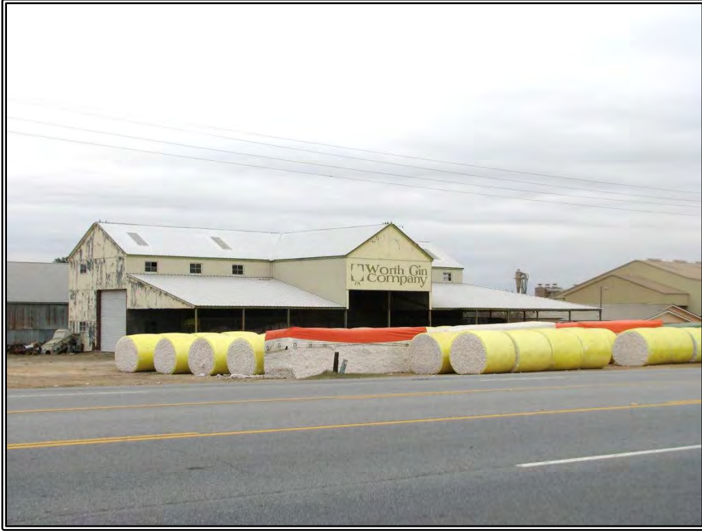
Photograph 14. View of Resource 4, circa 1960 main building, southwest oblique.
