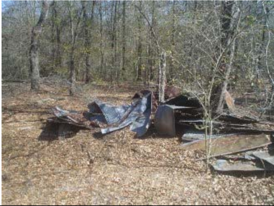
Photo 13: View of the remnants of a structure in the center of the subject property, facing north-northeast
