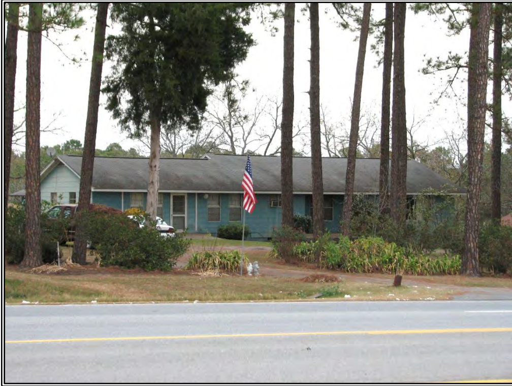
Photograph 17. View of Resource 5, south front elevation.
