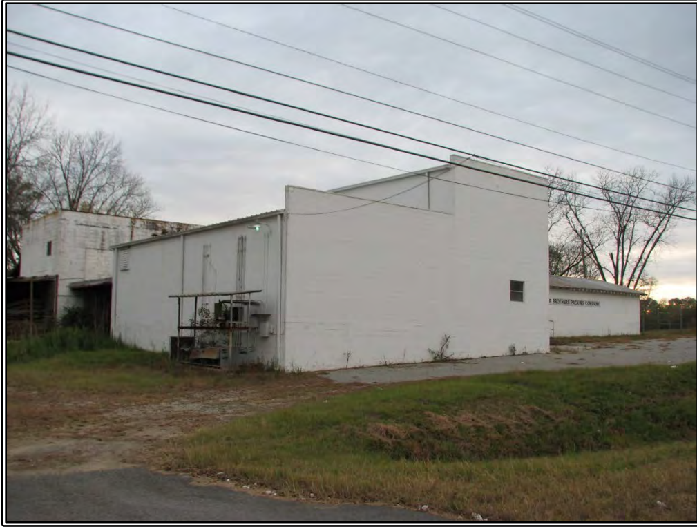
Photograph 20. View of Resource 6, circa 1970 addition, northeast oblique.
