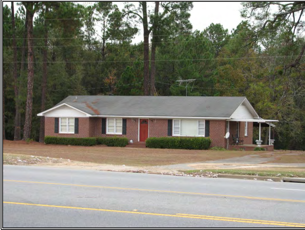
Photograph 13. View of Resource 3, south front elevation.
