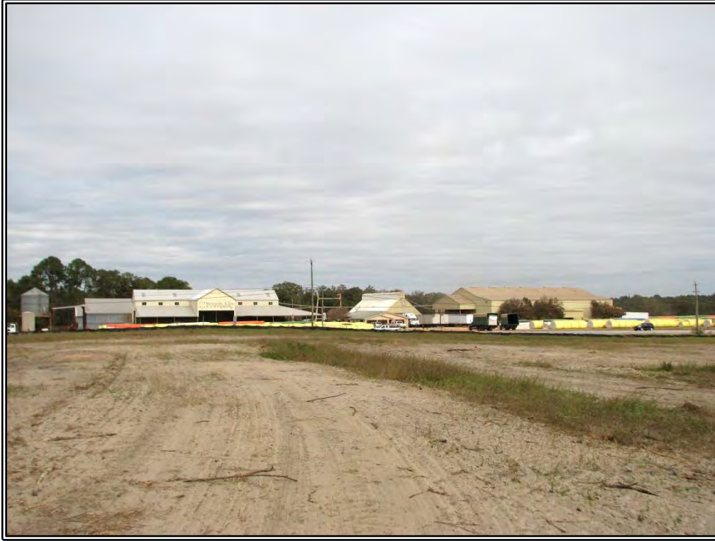
Photograph 16. View of the Resource 4 complex, looking north from the project tract.
